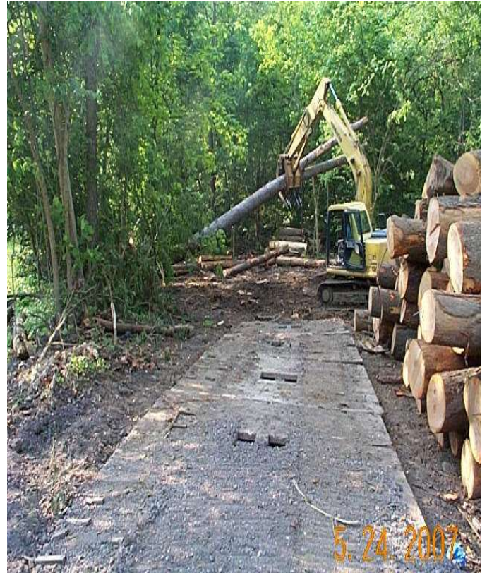
Above photo: Mud Mats installed at landing site
